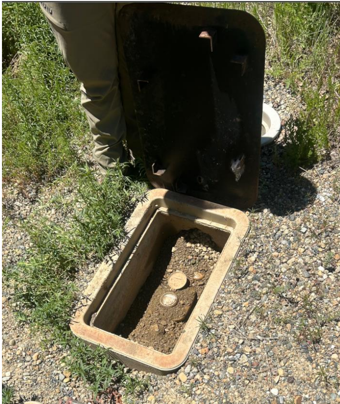
Figure 2-4. Water meter located within a concrete vault; periodic observations of these were recorded to track applied water volumes over time.
