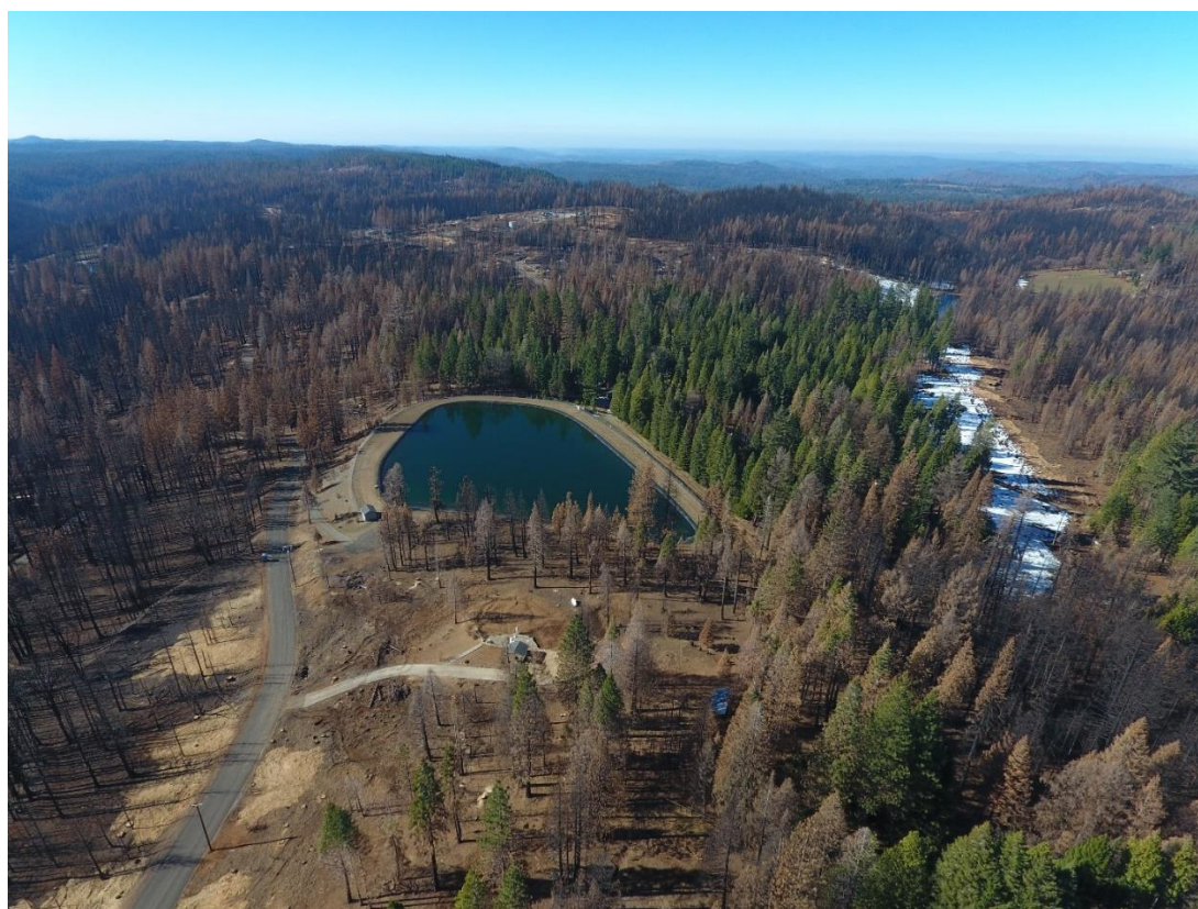
Figure 2. Wildfire Damages near Facilities of Grizzly Flats Community Service District (January 20, 2022) (Courtesy from Grizzly Flats Community Services District; copyright reserved)
