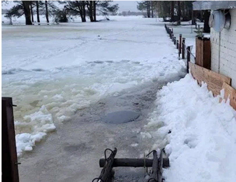
Upper Truckee Meadow floodwaters flowing toward STPUD's pump station during large March 2023 rain-on-snow event.
