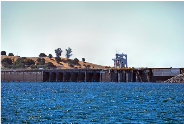
Folsom Dam and reservoir (USBR/Winetta Owens)
